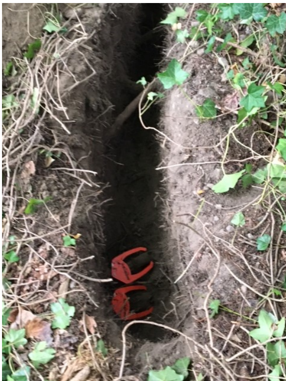
Photo 1 A . Trench near Tree #214. 8' long, 22" deep. Very few roots
