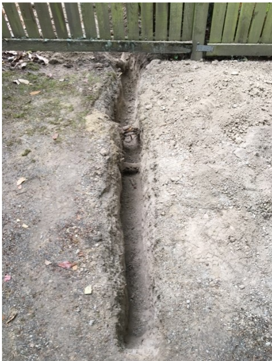
Photo 6. Tree #227 trench looking south
